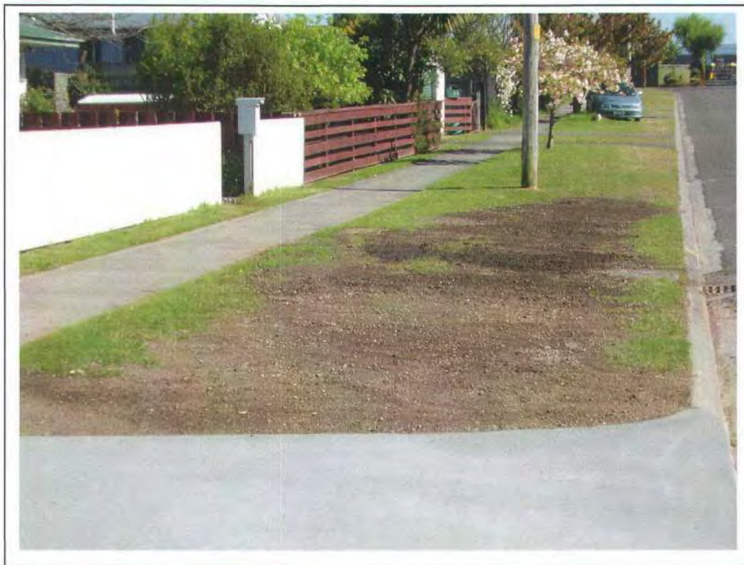
Photo 2 – Levelled Berm and Reinstated Kerb
