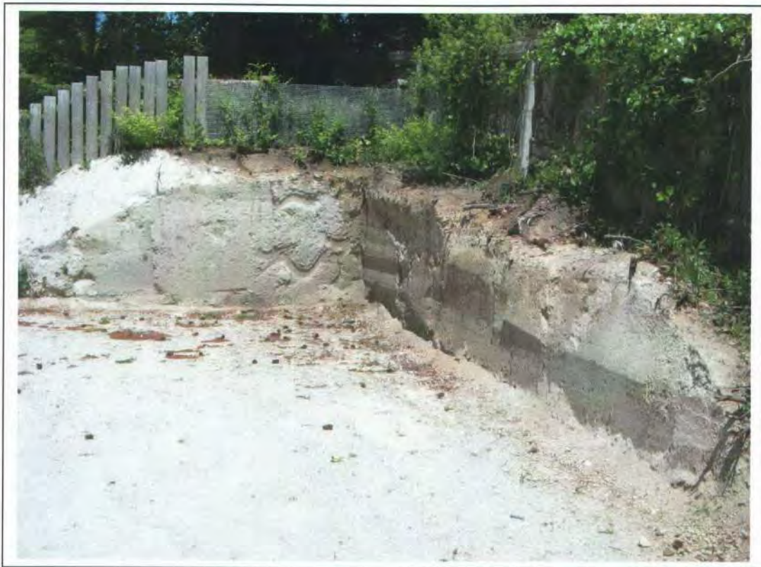
Photo 2 – Vertical cut on south western boundary (EW 1 and 2).
