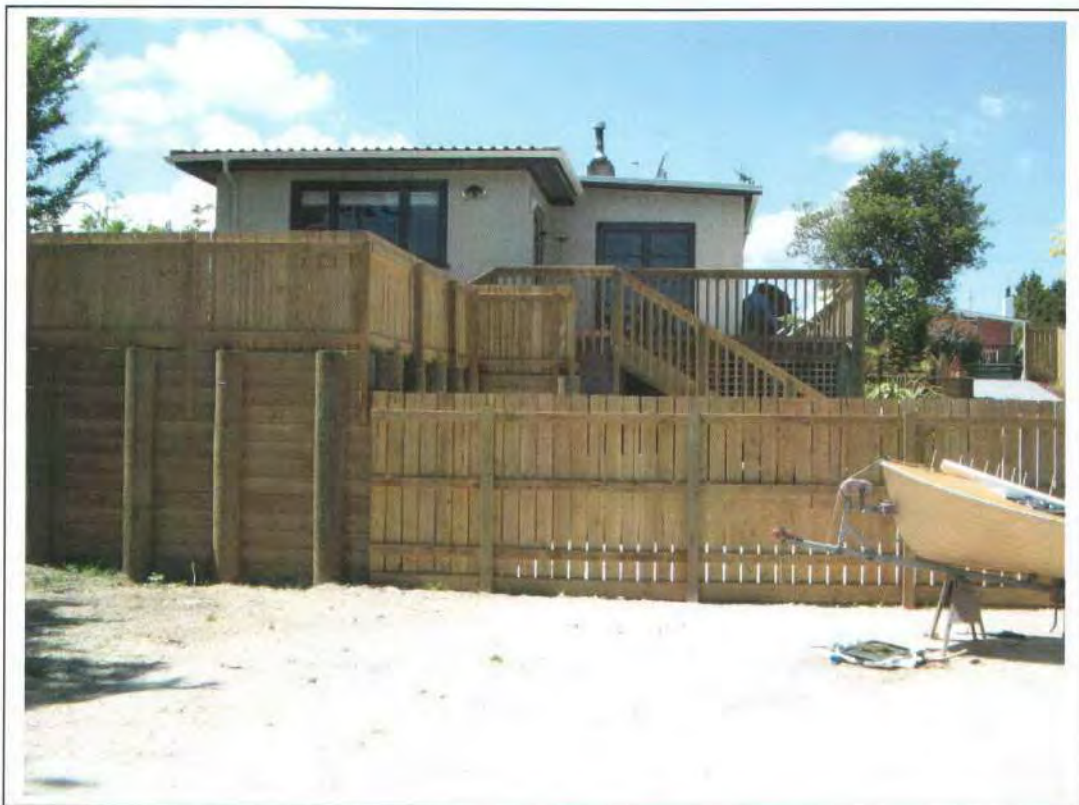
Photo 6 – Retaining wall (RW 2) on north eastern boundary.
