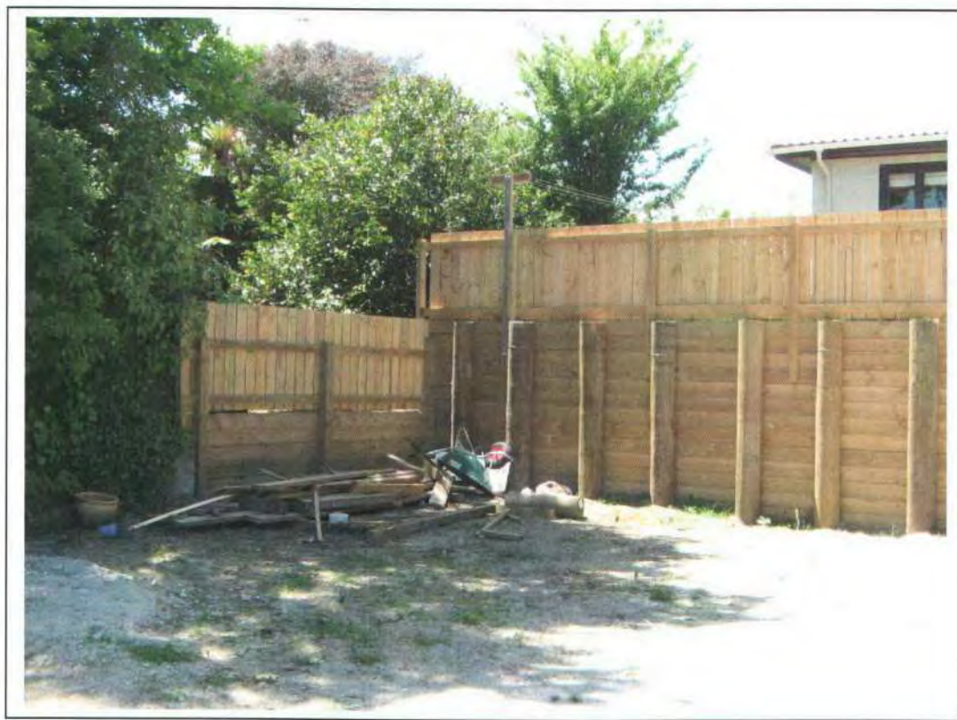
Photo 5 – Retaining walls at north eastern corner of Lot 2 (RW 1 and RW2).
